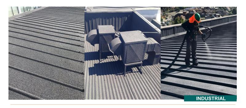
**Isolcork** Sprayed Rubber combines waterproofing and recycling. It is formulated with 100% recycled rubber from used tires. It allows to form a continuous membrane in a fast and safe execution.
